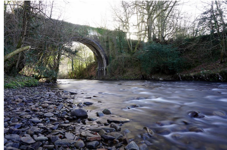
Figure 5: Penllwyn Tramroad Bridge, Nine Mile Point
