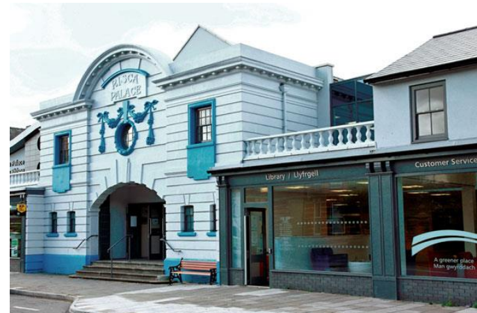
Figure 2: Former Palace Cinema, Risca
