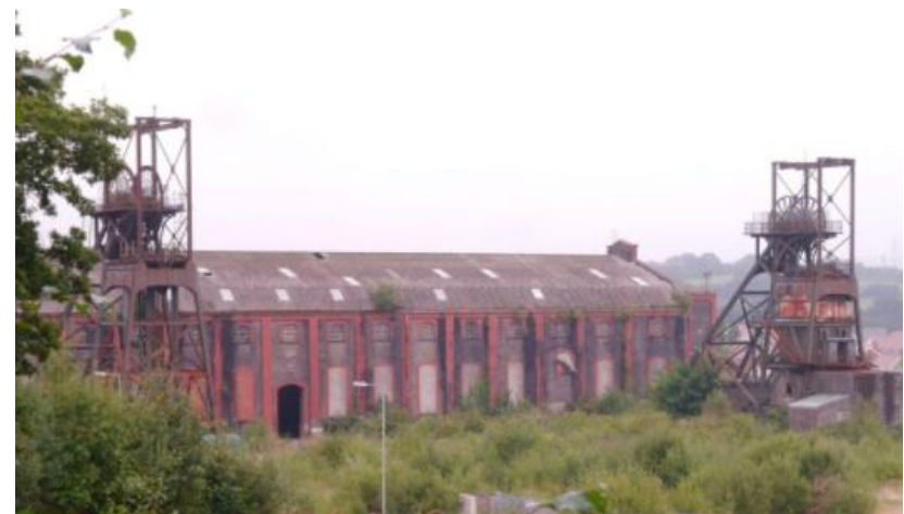
Figure 8: Penallta Colliery Engine Hall & Fan House, Ystrad Mynach
