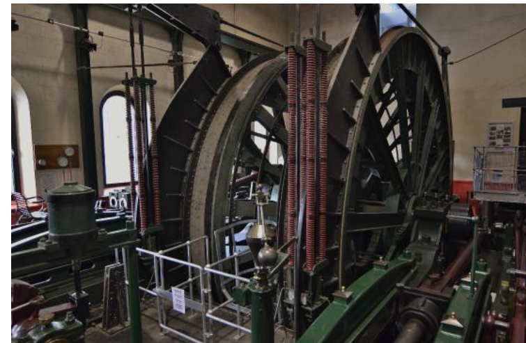
Figure 2: Winding House Engine, New Tredegar
