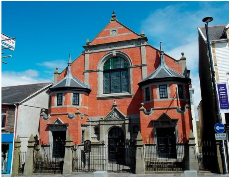
Figure 7: Hanbury Road Baptist Chapel & Schoolrooms, Bargoed
