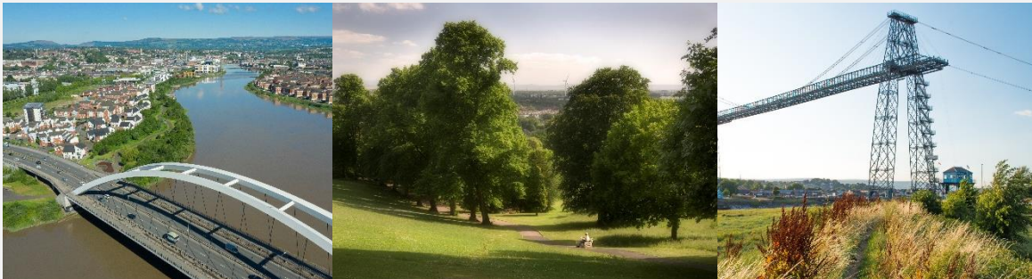
Figure 9: (Left to right) Southern Distributor Road Bridge in Newport, Beechwood Park, Newport, and the Transporter Bridge.
